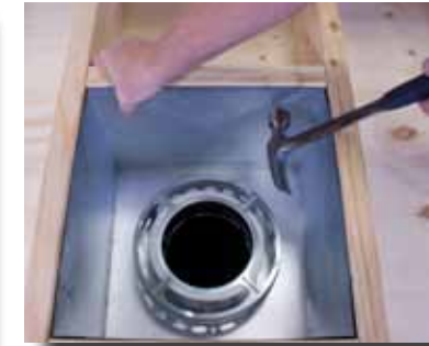
3. Nail the chimney support box to the framed opening from above. Use at least two 8 penny nails on each side.
