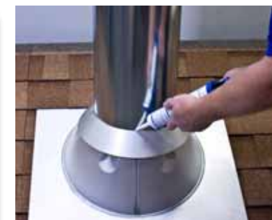
13. Apply high temperature silicone sealant where storm collar will meet chimney. Slip storm collar around chimney and slide down. Seal with high temperature silicone sealant.
