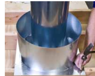
6. Slip insulation shield over chimney until base sits squarely on framed opening or nests in the support box. Nail to opening or screw to box.
