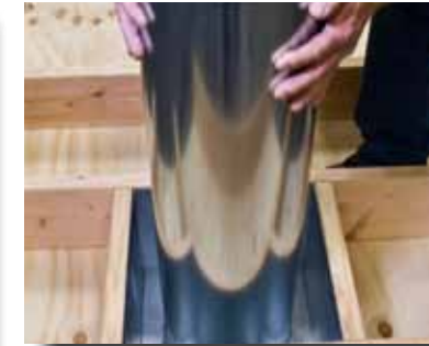
5. Lower the first chimney section over short piece of pipe in the bottom of the support box. Push together and twist to lock.
