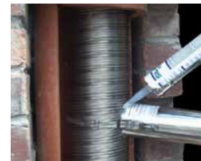
8. Fasten and seal Universal Take-off to VENTINOX.
