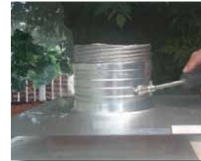
5. Secure VENTINOX on top with Top Plate and Storm Collar.
