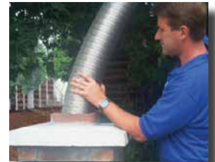
3. Insert VENTINOX into chimney.
