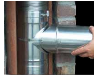
4. Feed liner through Snout's drawband, then fasten.
