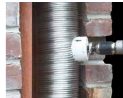
7. If needed, cut Universal Take-off hole into VENTINOX.
