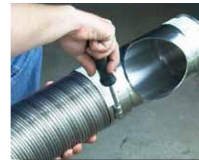
2. Secure Tee body with Tee Cap to liner.
