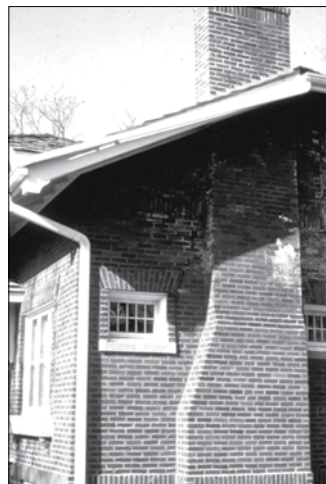
Spalling bricks
